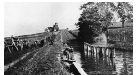
Plane 9 West, the longest and highest plane on the Morris Canal, was 510 feet long to its summit and 1,788 feet long from end to end. It was one of three planes with a double set of tracks.
